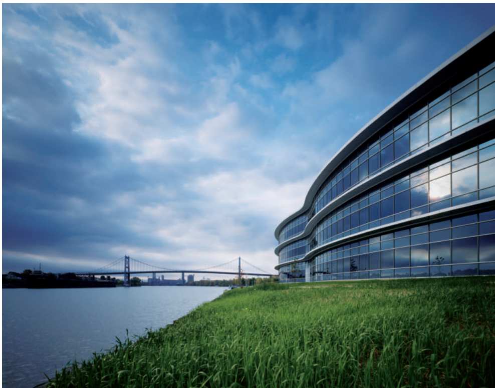
Owens Corning World Headquarters, Toledo, OH; provided courtesy of Owens Corning
