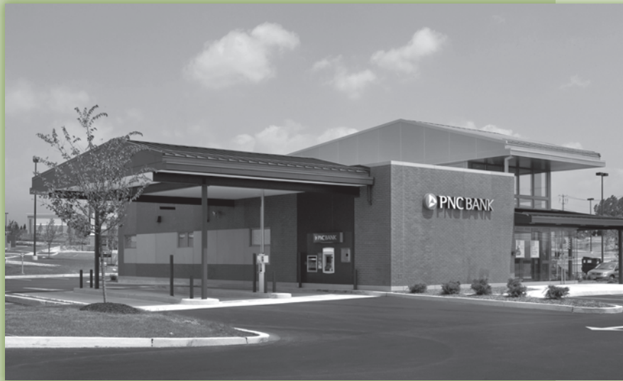
PNC Bank's green prototype in East Bradford, Pa., is a 3,650-sf branch that was constructed in the shortened 4-6 week construction period of all of PNC's volume LEED certified green branches.
