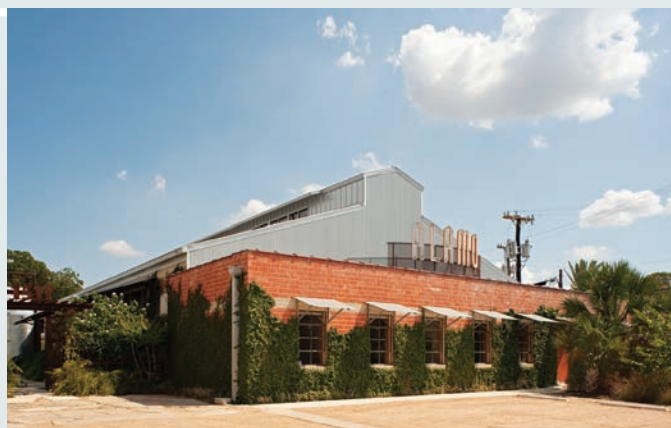
SoFlo Office Studios, San Antonio, TX
